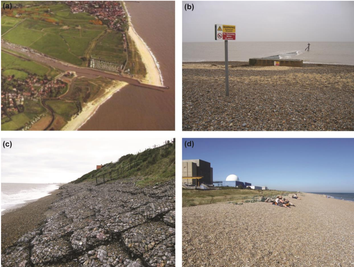
Figure 2: Coastal 'hard points'. Formed by (a) the entrance piers to the Blyth estuary, (b) Minsmere sluice, (c) Coralline Crag sub-crop and coastal defences at Thorpeness; photograph (d) shows the beach and artificial dune defences in front of Sizewell 'A' and 'B' power stations.
